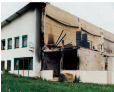
A fatal fire destroyed the factory floor. Thanks to the THERMODUR firewall the bureaus remained unaffected.
